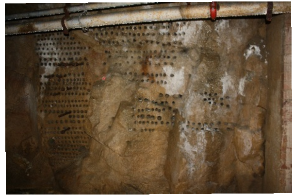
Photo:- Test holes drilled by Holmans
