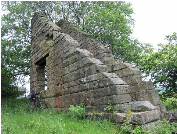
Photo:- Railway Pit coke ovens structure
