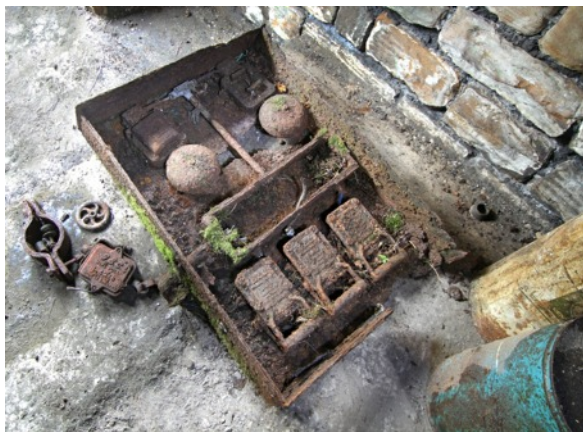
Hemingfield Colliery Pumping Shaft Banksmans Controls -Image by David Kitching
