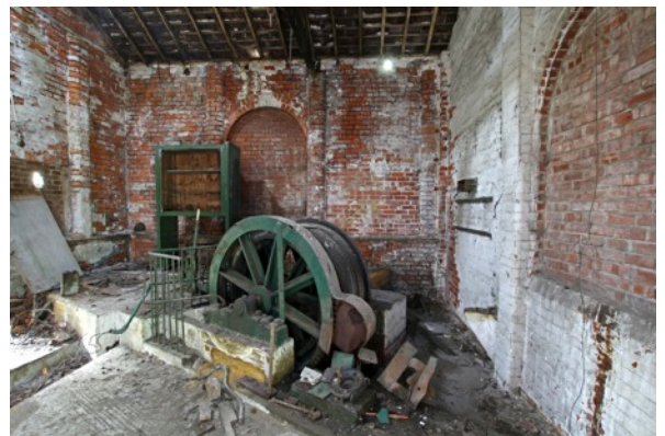
Hemingfield Colliery Winding Engine-Image by David Kitching
