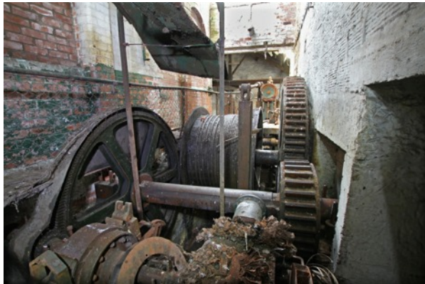
Hemingfield Colliery Winding Engine-Image by David Kitching
