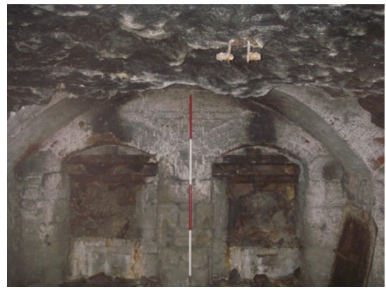
Photo:- Twin drawholes in one of the tunnels
