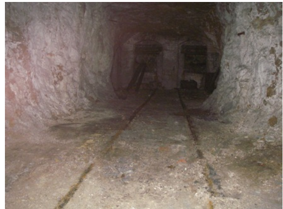
Photo:- Rail track in situ in one of the tunnels
