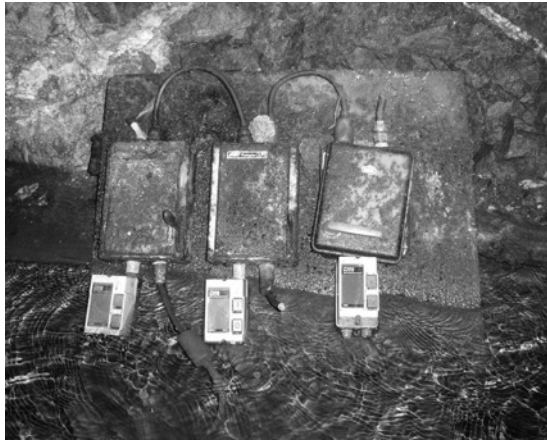
Photo:- Electrical switchgear
