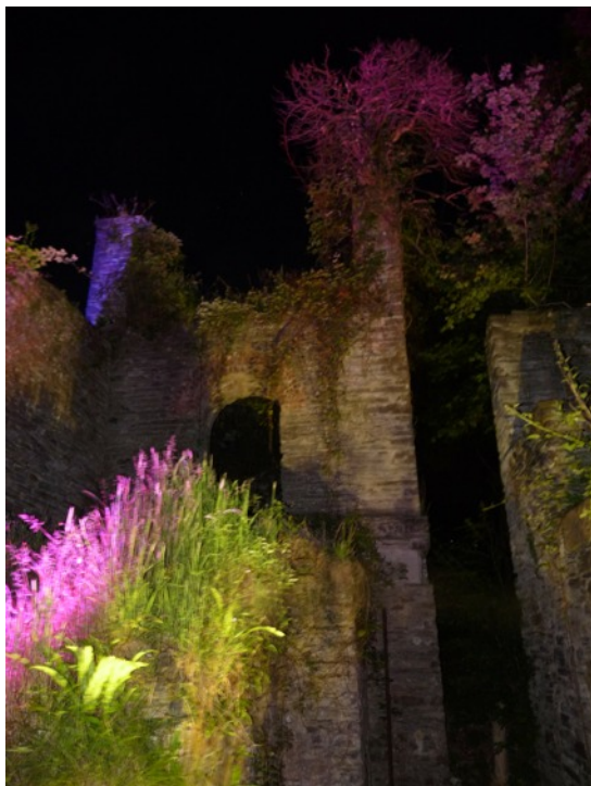
Photo :- The engine house
