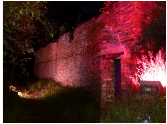
Photo :- The boiler house
