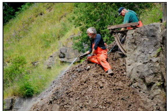
Photo:- Under careful scrutiny from above, a powerful stream of water cleanses the material just tipped from the wagon
