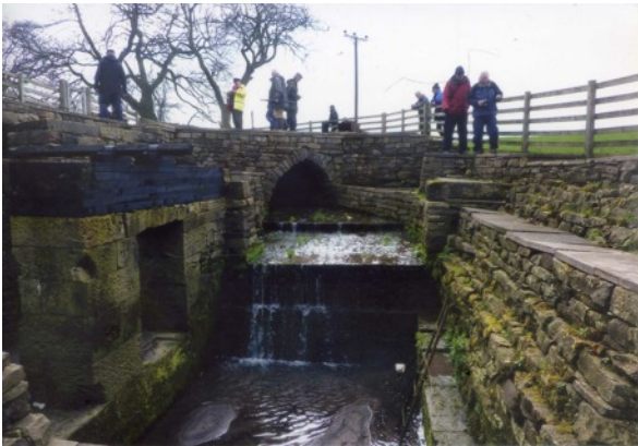
Photo 1. Worked with a 12' dia waterwheel, a 6' dia cog wheel turning a 12' drum.
