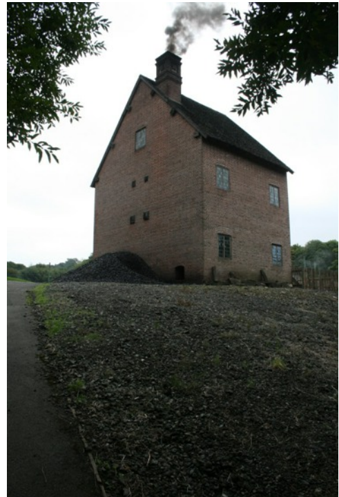
Photo:- The engine house
