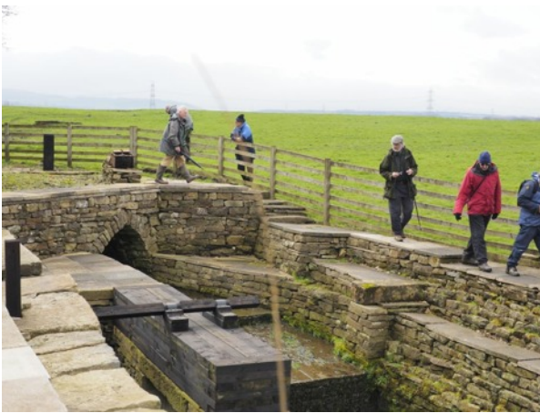
Photo 2. Dunkirk Mine Haulage Water Wheel Foundations Rebuilt by Richard Matthews & Brian Jeffries
