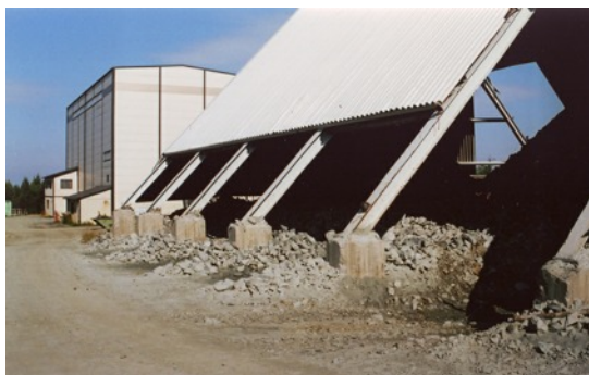
Photo:- Exterior of the mill
