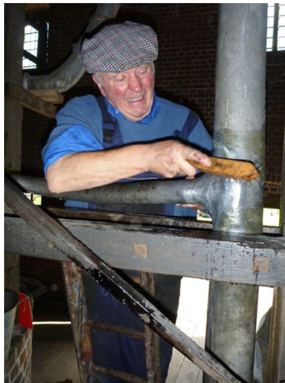
Photo:- wire brushing the joints clean
