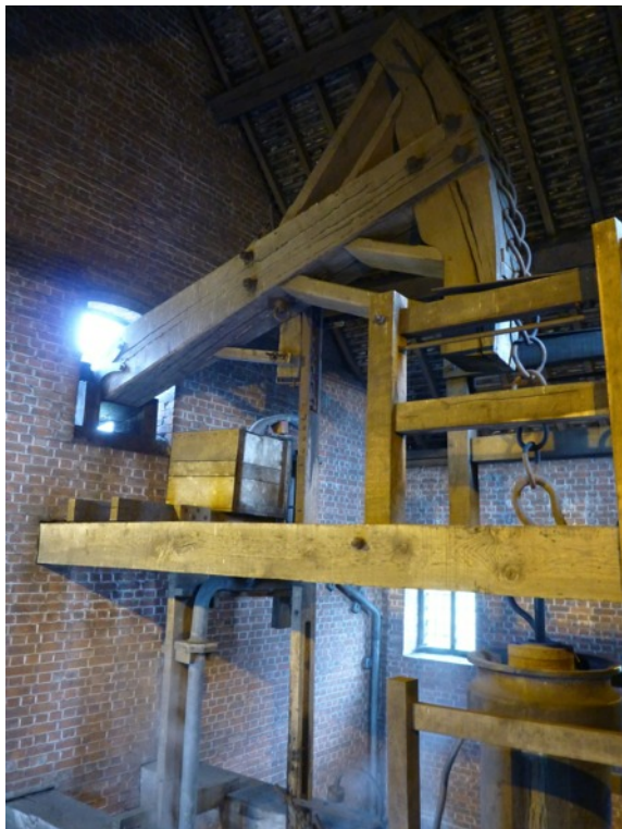
Photo:- Indoor Beam end and Archhead
