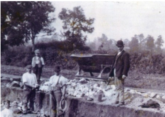
Photo: Early V-tipper wagon in use at celestine workings, near Yate
