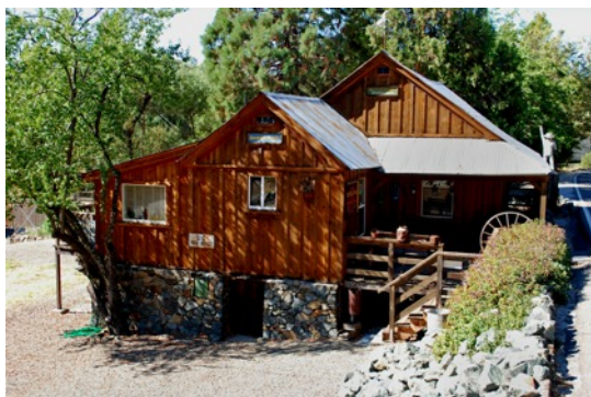
Photo: Old toll house
