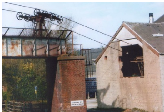
Photo 2. View of the building next to the A683 Hornby to Lancaster road. Seen in April 2008, this year the building has been totally re-roofed, this being the start and return of the newly-painted buckets.
