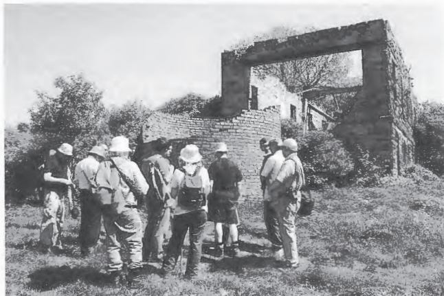
Group at the downcast shaft and combined winding and pumping house.
