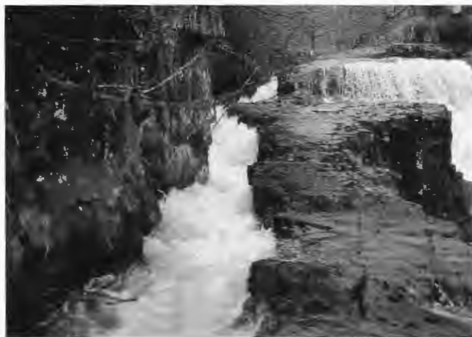
The channel that ducts water from the waterfalls of the Afon Gain (to be seen on the RHS) to the former waterwheel at Tyddyn Gwladys
