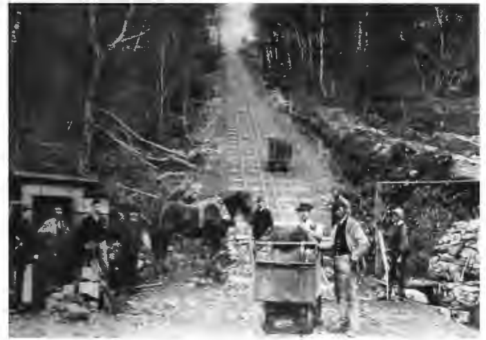
A restored 19th century photograph showing the hoist, which transferred bogeys from the upper levels to the main level of Gwynfynydd gold mine. Now overgrown, the feature is very hard to detect.
