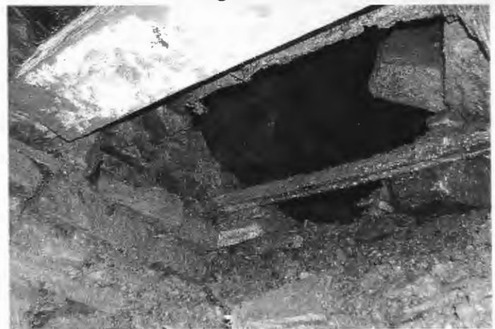
Access to the top of the Dig
