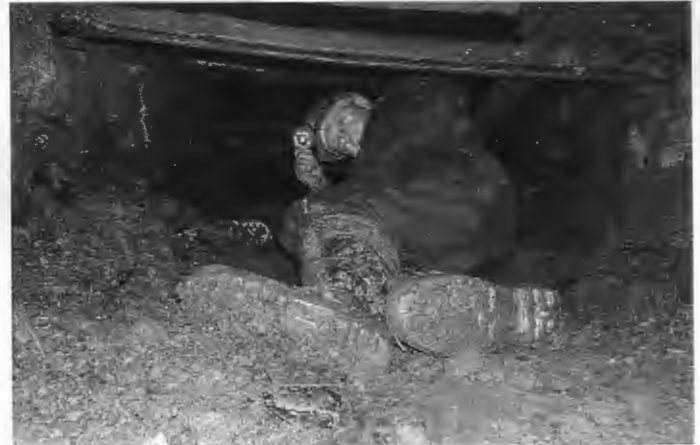
Archie Meadowcroft inspecting the work
