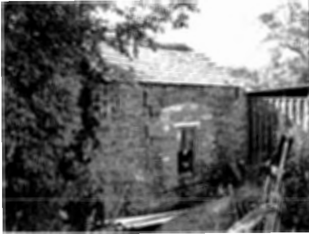
Photograph 1 Constructed of red brick marked Claughton, the building details are as follows; 140 in length, 90 in width. Height to gutter level 96. Original window 60 x 56. Unseen external door 70 x 26. A standard gauge 48½ railway ran alongside the window.
