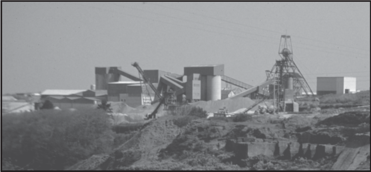
New Cooks Kitchen Shaft, South Crofty. (Mike Gill, 1976)
