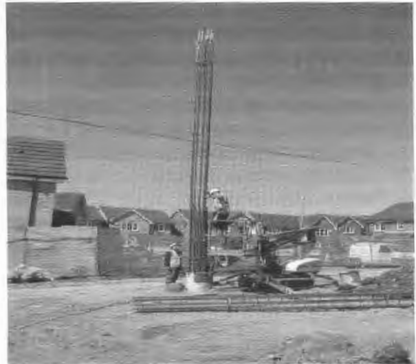
Assembling the steel piles on the ground, and with the aid of a tall crane the piles were lowered into the pre-drilled holes
