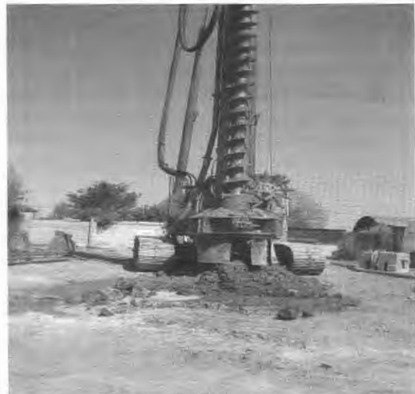
The CTA drilling machine is digging one of the 68 holes. The holes are precisely dug with the aid of an onboard computer and monitor located in the cab.
