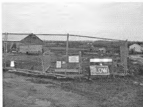
Croft Side Colliery Air shaft collapses for the second time in 3 months.
