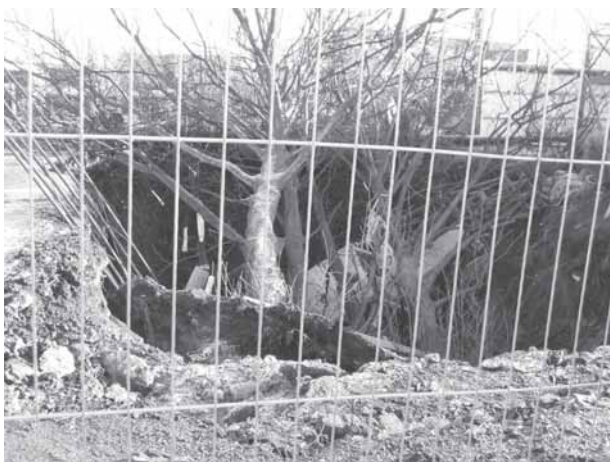
Shaft collapse at Darcy Lever Photo by Adrian Turner
