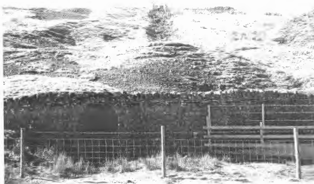
Hunt's Coldberry level portal with water balance incline above
